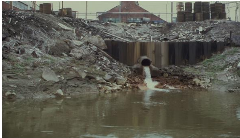
Plate 2. An outfall or discharge point at Unilever Plc is a common practice by industries in major cities in Nigeria.
